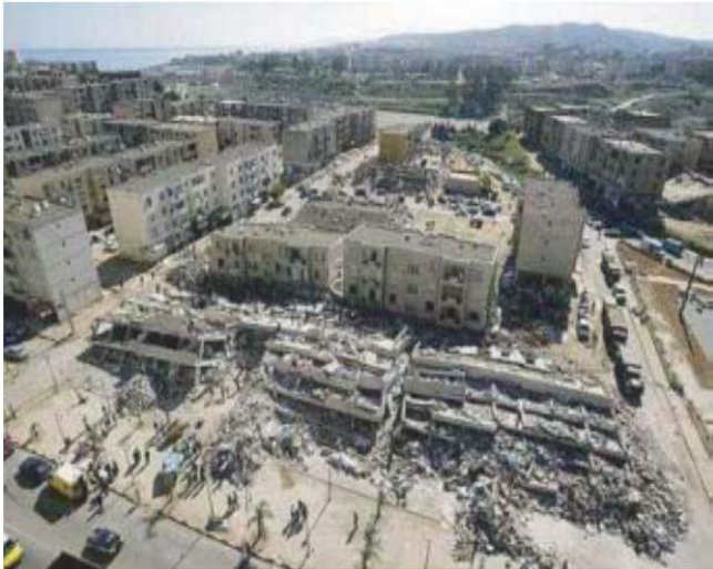
Fig. 2 Building damages observed in the city of Boumerdes (photo from CSEM-EMSC September 2003)
