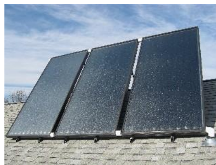
Fig. 1 Flat Plate Collector
